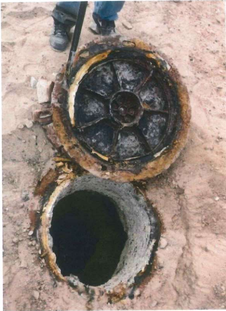
Two additional Pre cast concrete manholes with major corrosion
