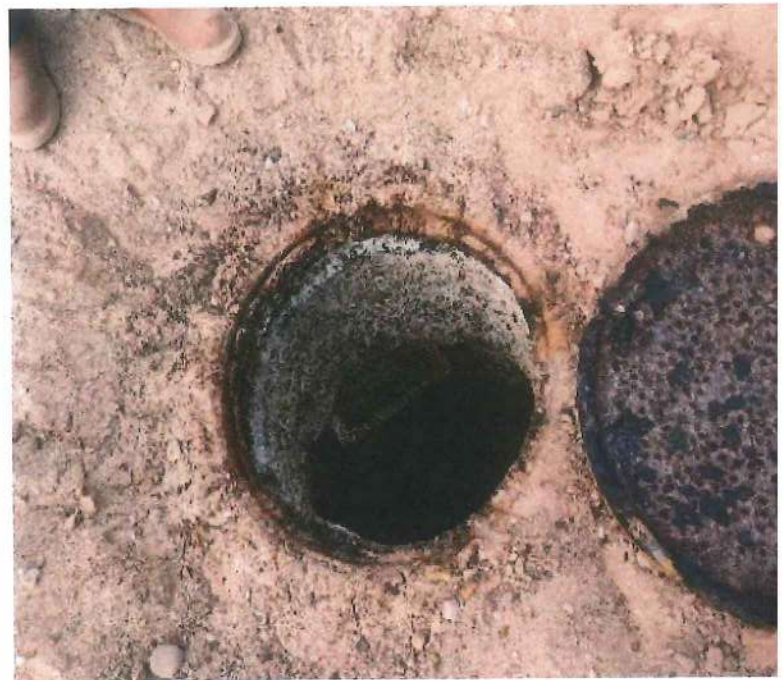
Two additional Pre cast concrete manholes with major corrosion
